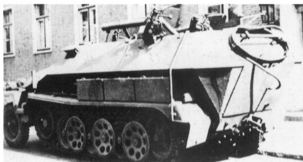
A flamethrower system similar to that developed for the Panzerkampfwagen B2 (F) was modified for mounting in the mittlerer Schützen-Panzer-Wagen Sd.Kfz.51 Ausf.C (medium armoured personnel carrier) from January 1943. This Flammpanzerwagen was designated Sd.Kfz.251/16. (Author)
